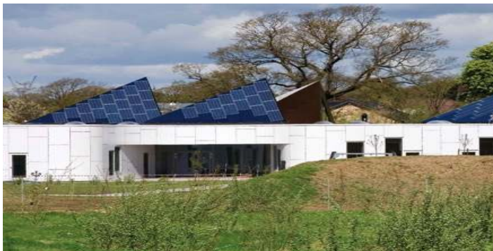
Solar panels on the roof of the kindergarten ©Cebra.dk
