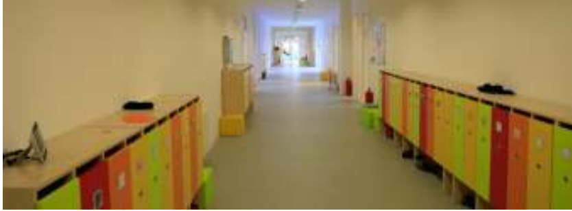
Rather wide corridor in width of one container module (2,4m).
